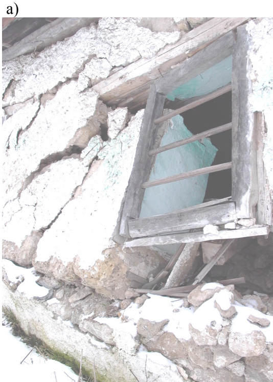
Figure 5: Northeast façade extracts a) scope of destruction at critical position, b) a closer look to the masonry and timber lacing
