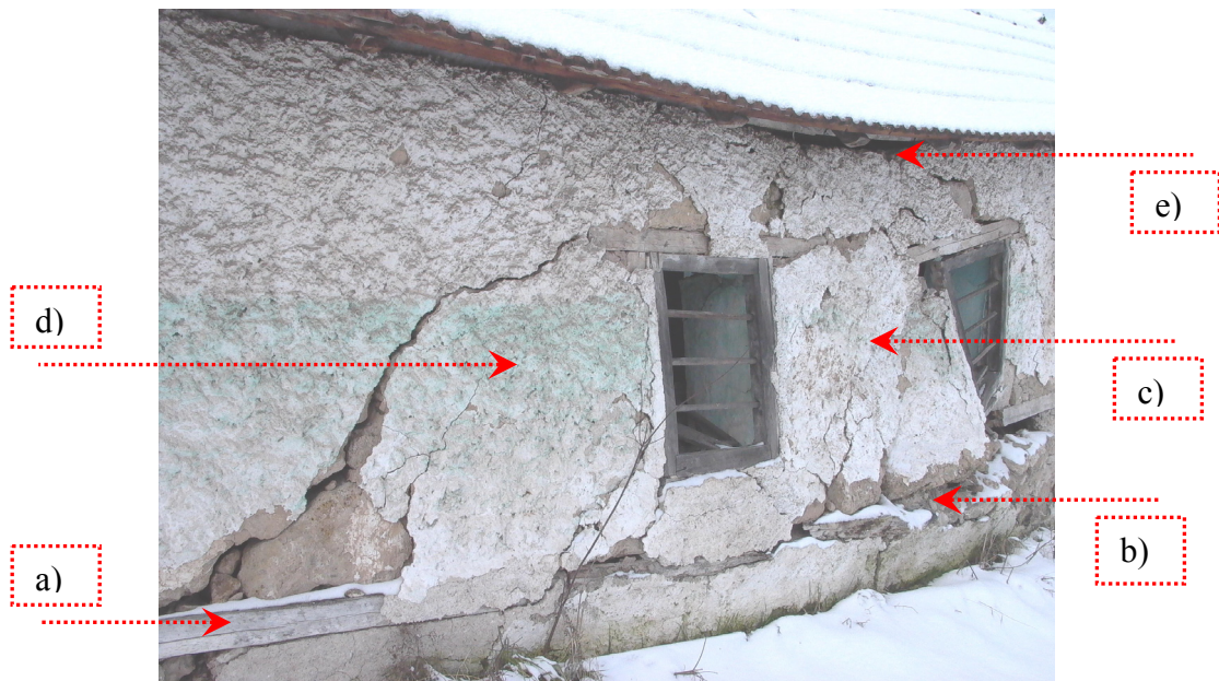
Figure 4: Northeast façade, extract a) timber lacing (outer joist) at approx. mid height of the building, b) timber lacing missing outside and decayed inside, c) overturned masonry block assemblage between the windows, d) the next endangered masonry block assemblage, e) masonry settlement, top timber lacing and eaves deformed
