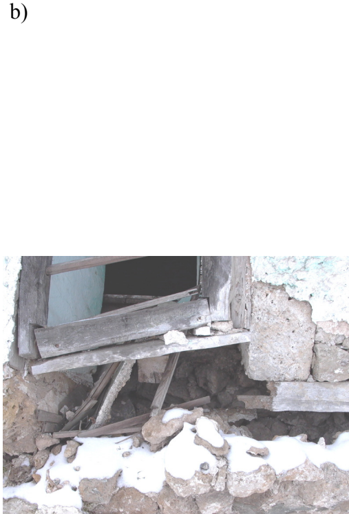
Figure 5: Northeast façade extracts a) scope of destruction at critical position, b) a closer look to the masonry and timber lacing
